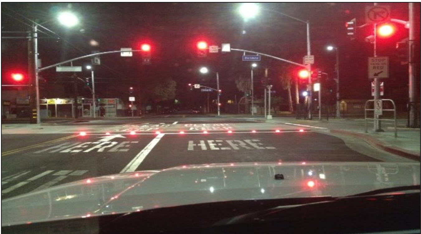
Marking this dedicated busway, the red in-roadway warning lights are directly in the line of sight creating a visual barrier, focusing the attention of the driver
